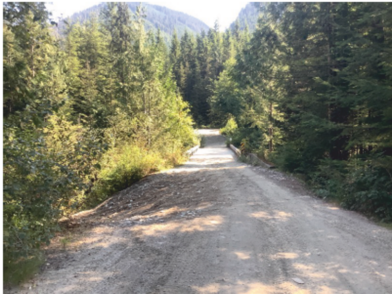
Right Bank Abutment when facing downstream
