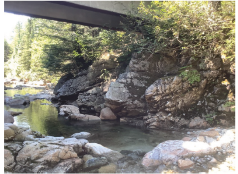
Right Bank Abutment when facing downstream
