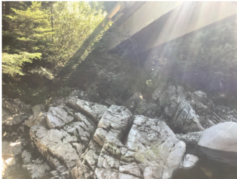
Left Bank Abutment when facing downstream
